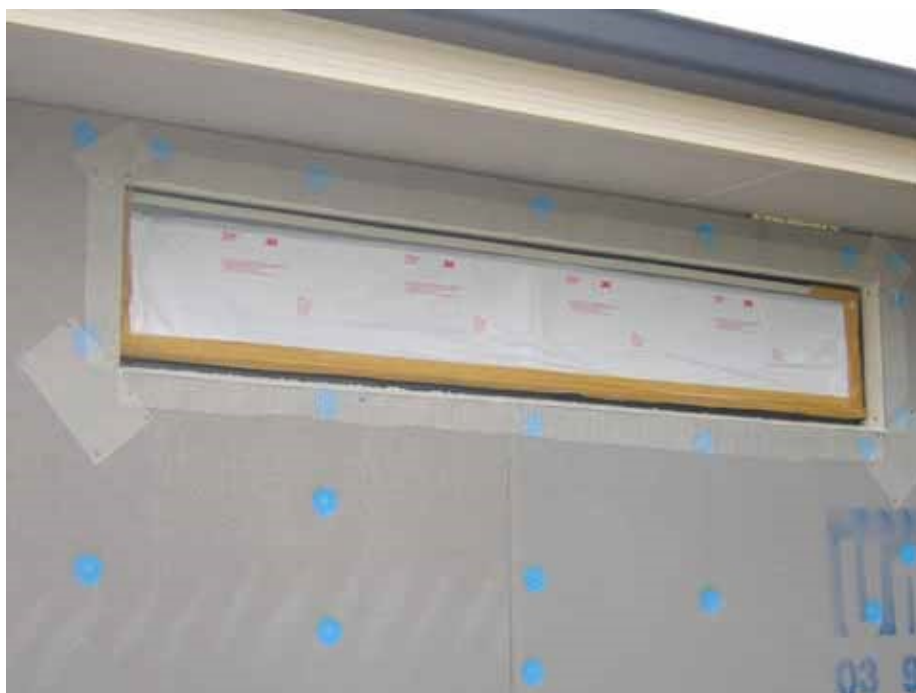
Fastener Positioning Details
